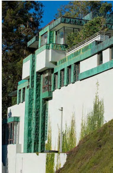
31. Samuel-Novaro House, Los Angeles
