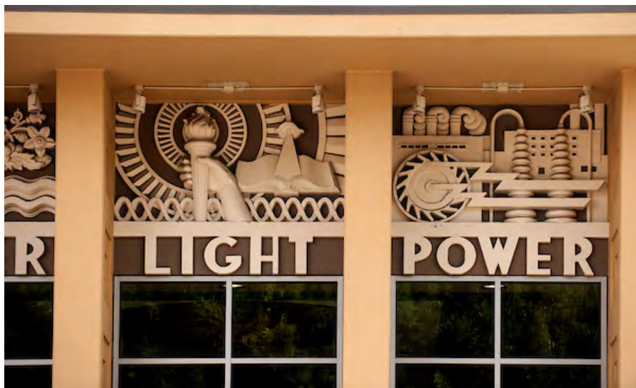
46. Burbank Water and Power, Exterior Detail, Burbank
