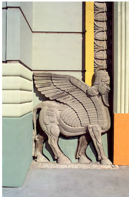
24. Samson Tyre and Rubber Company, Exterior Detail, Commerce
