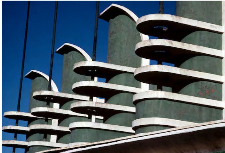
21. Pan Pacific Auditorium, Exterior Detail, Los Angeles
