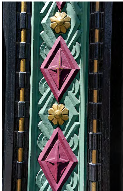
56. Rowan-Bradley Building, Exterior Detail, Long Beach
